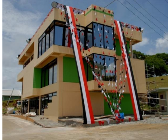
Works Head Office Extension
