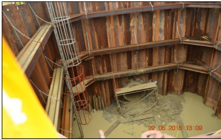
Receiving Shaft of Tunnel – Malabar Plant
