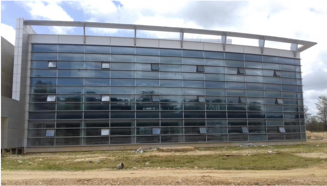
East Block Building 1 Eastern side
