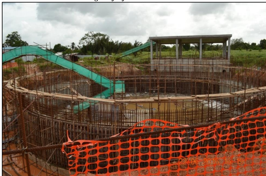
Storm Tank at Malabar Site
