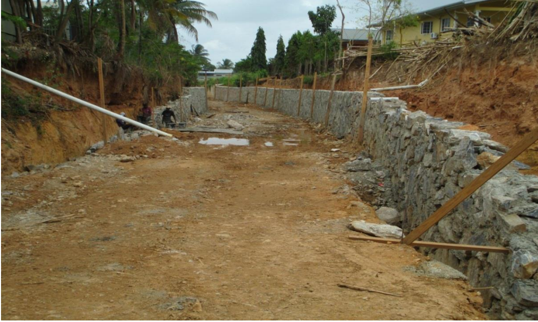
Rubble Masonry Wall at Miss Gutter Ravine - Five Rivers, Arouca
