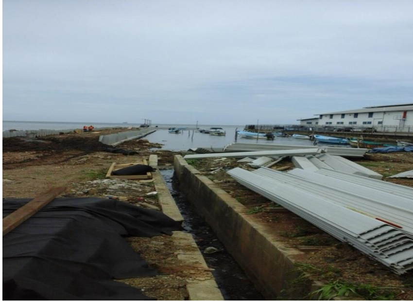
Construction of Slipway at Cocorite Fish Landing Facility
