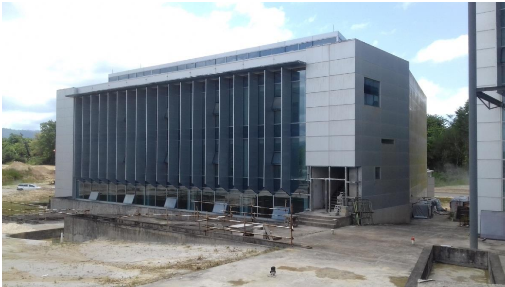
East Block Building 1 Western side
