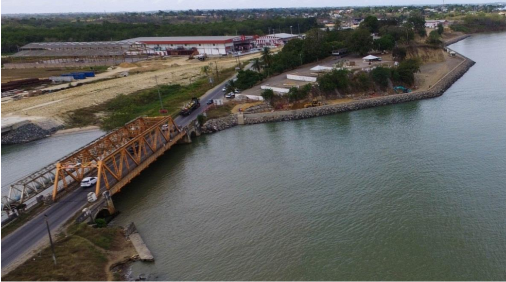
Aerial View of the Shore of Peace Cliff Stabilization Works –Mosquito Creek
