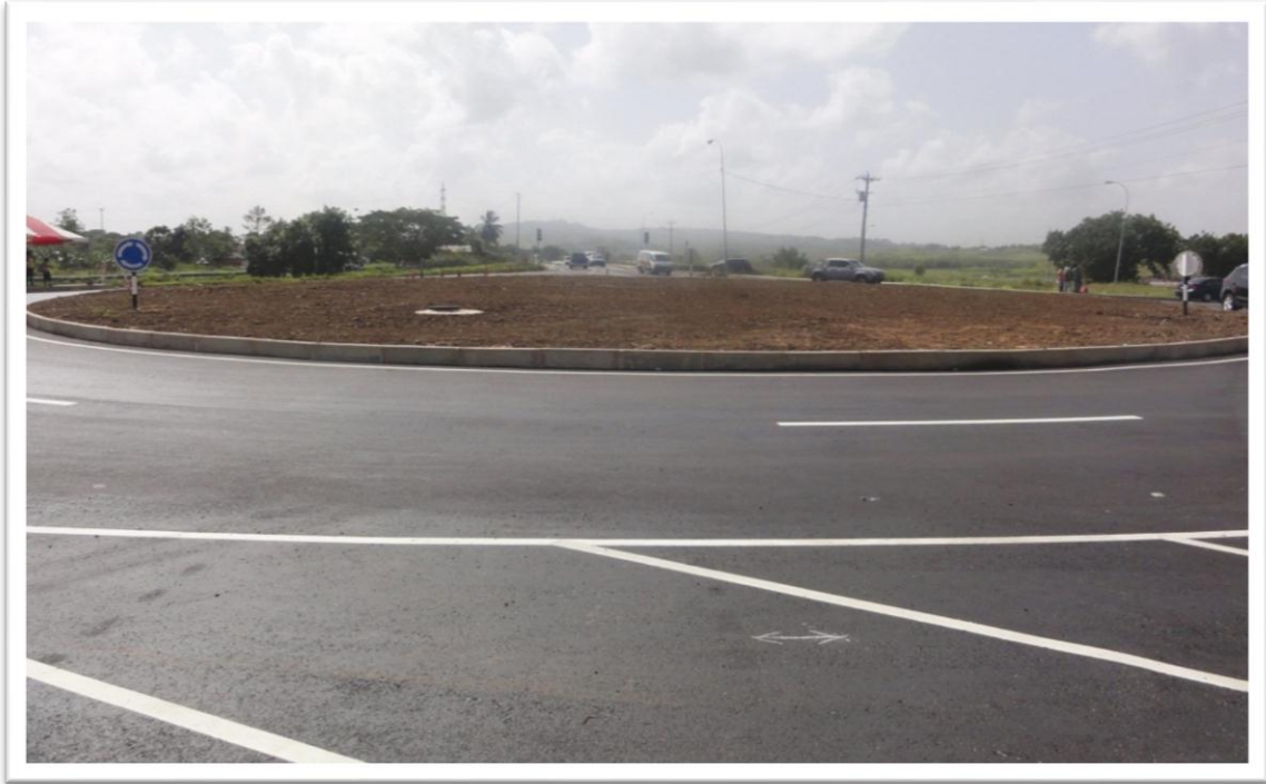
Couva Interchange - West Side North Roundabout
