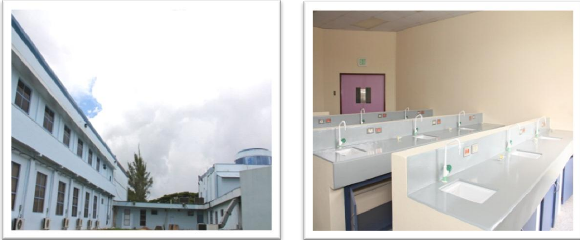
Upper East Wing Cipriani Labour College Exterior view and Laboratory
