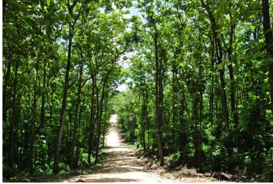
Forest Access Road in need of Rehabilitation
