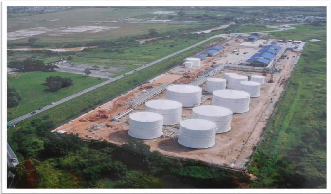
MultiFuel Pipeline Storage Facilities at the Blue River Interchange, Caroni
