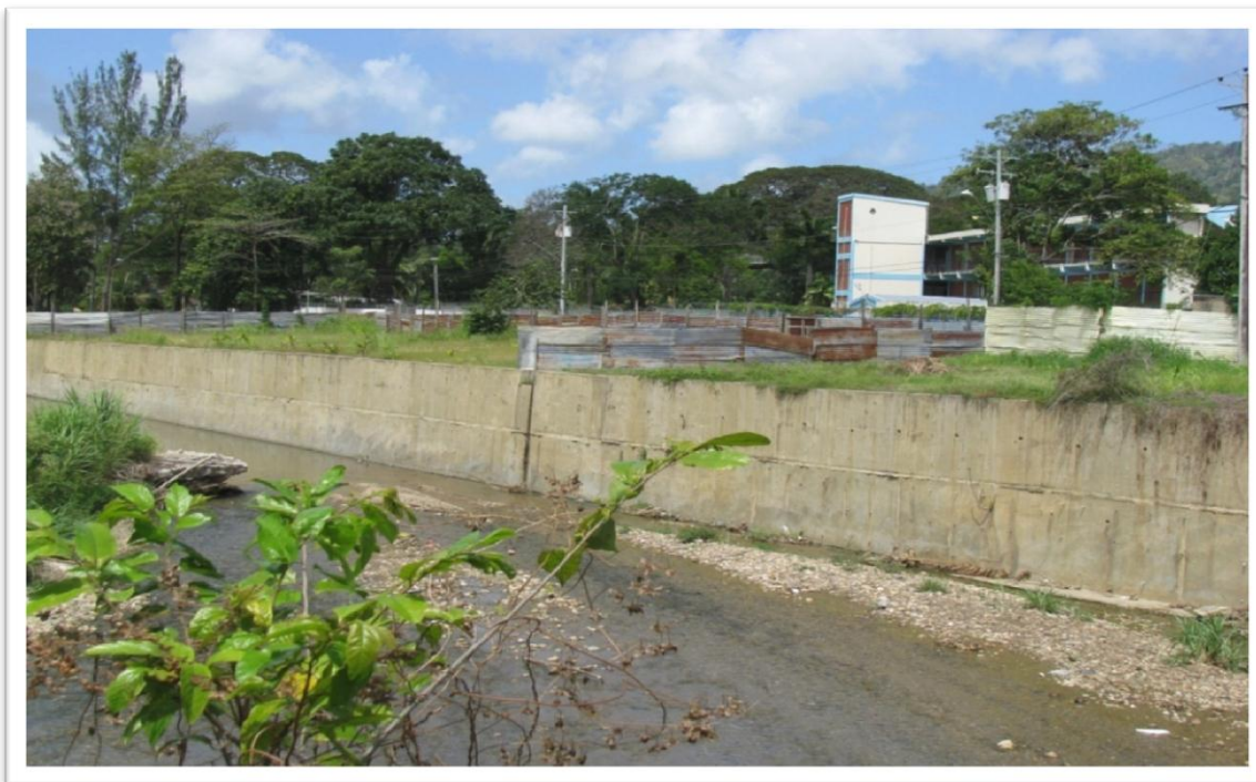
Reinforced concrete wall constructed on the St. Joseph River at Site 3 Farm Road
