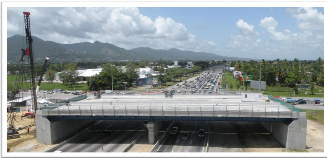
Bridge Construction at the Churchill Roosevelt and Uriah Butler Highways
