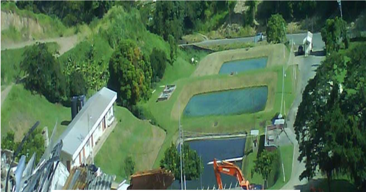
Studley Park Integrated Waste Facilities - Ponds for Liquid Waste
