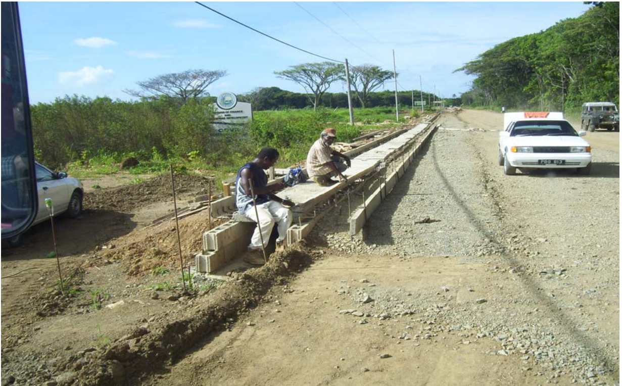
Cove Industrial Park – construction of access roads
