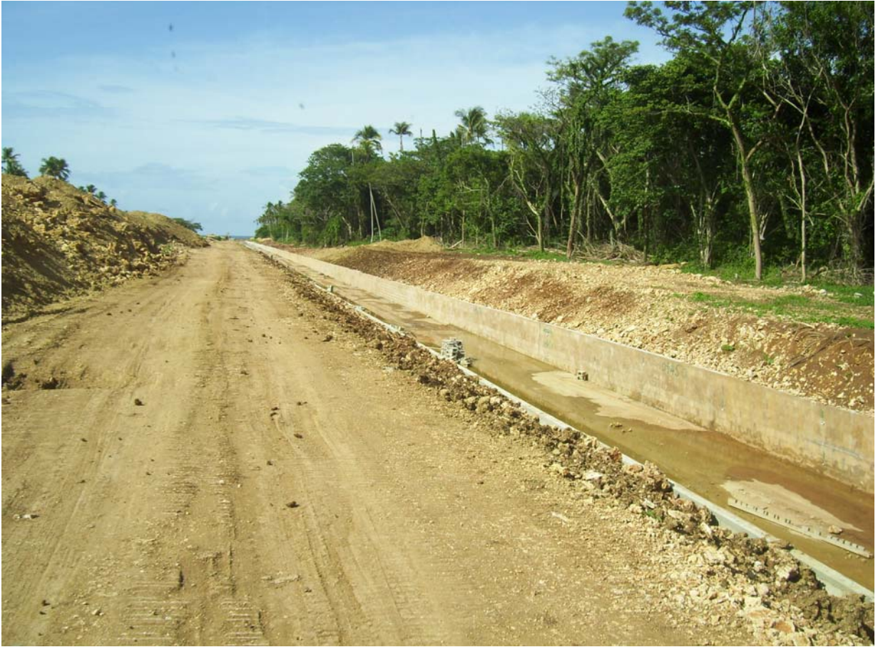
Cove Industrial Park – construction of outfall Drain
