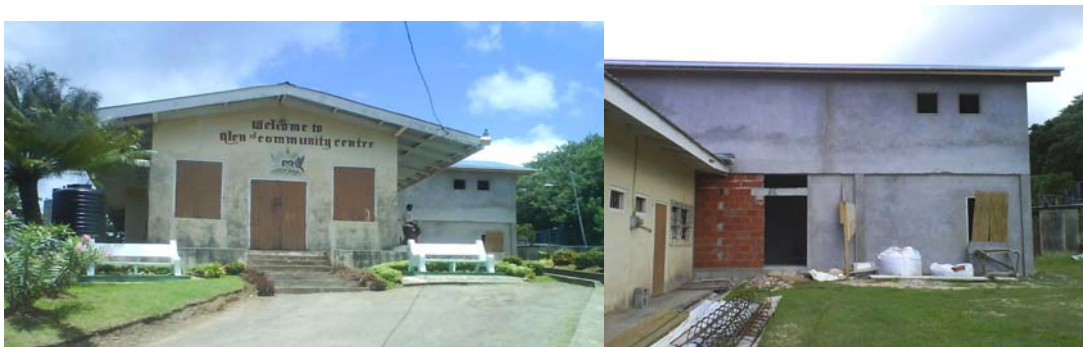
Glen Road Community Centre – Old section to be demolished, and new section under construction
