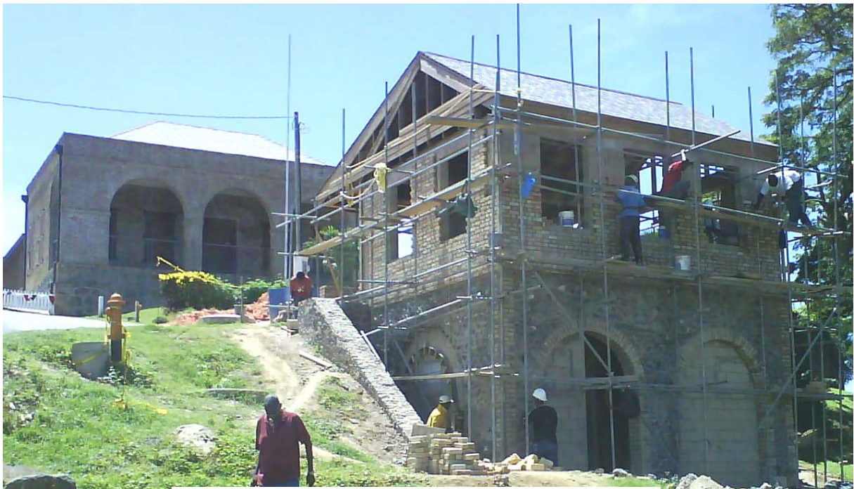
Fort King George Heritage Park – barracks being rebuilt
