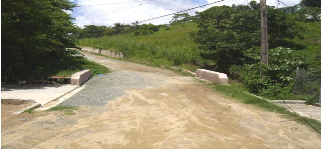
Streets of Plymouth – widening of roads
