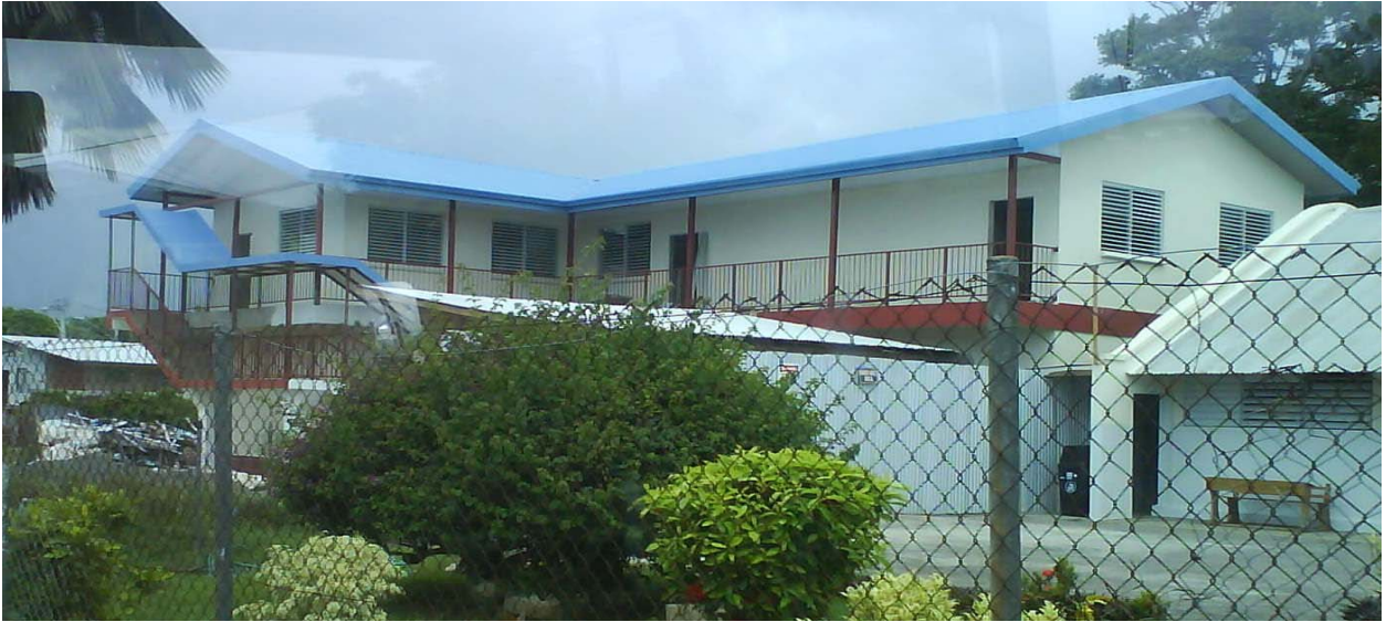
Plymouth Anglican School – Extension to the school
