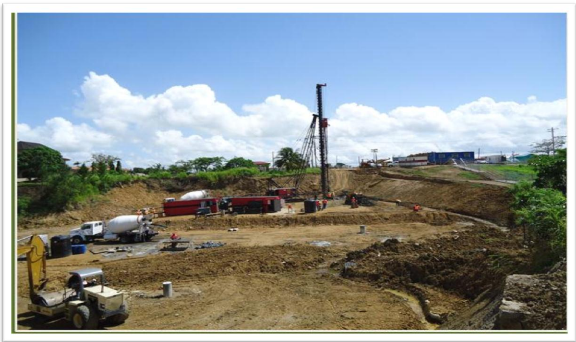
Construction works at B1/3 Calcutta Road No. 2
