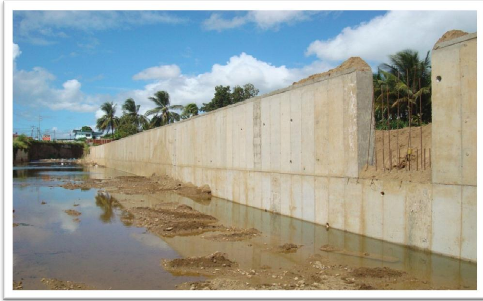
Construction of reinforced concrete wall on the north bank of the San Juan River
