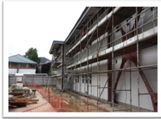
Arima Police Station
