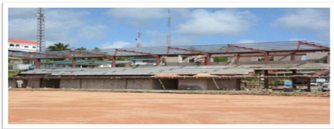
Yolande Pompey Recreation Facility Pavillion under construction
