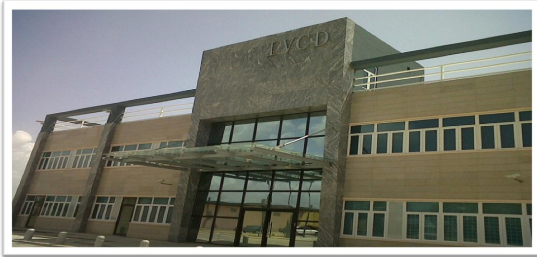
New Insect Vector Control Division Chemical Warehouse and Head Office Building
