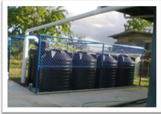
Rainwater Harvesting at Invernes
