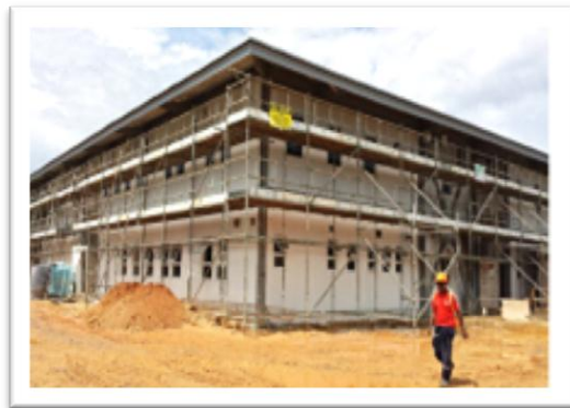
Piarco Police Station
