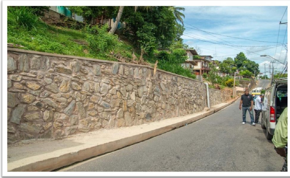
Retaining wall at Red Hill Morvant
