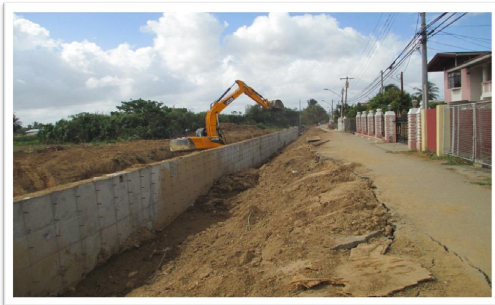
Tunapuna River Improvement Works – Dry River Trace
