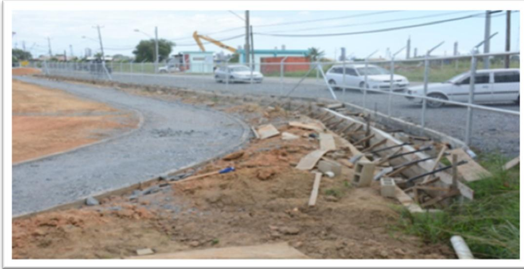
Phoenix Park Recreation Ground
