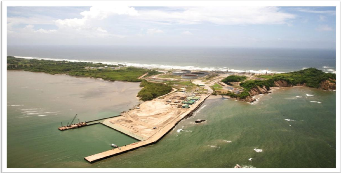
Overview of construction of the Galeota Port
