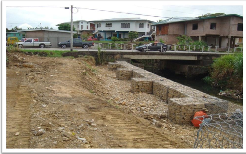
Construction of Gabion Basket Wall at Manicou River Arima
