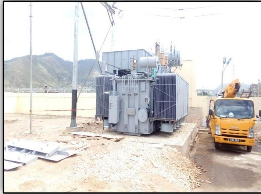
**100/130 MVA Transformer at Westmoorings Substation**
