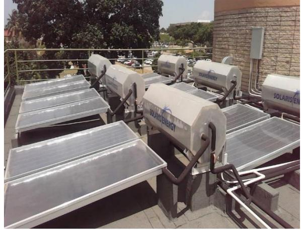
*Solar Powered Panels providing hot water to the Hall*
