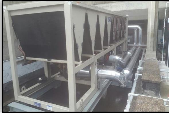
*Supply and Installation of a 295 Ton Air-Cooled Chiller System at the Riverside Plaza*
