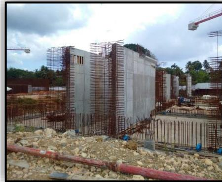
*Construction of Baffle Walls for Bioreactor at San Fernando WWTP*
