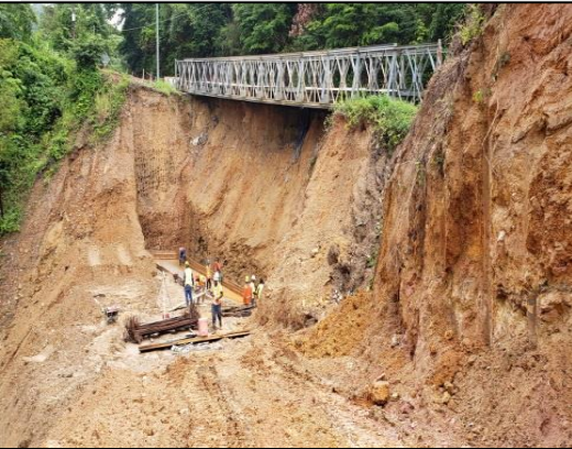
North Coast Road Slope Stabilization (11km Mark)
