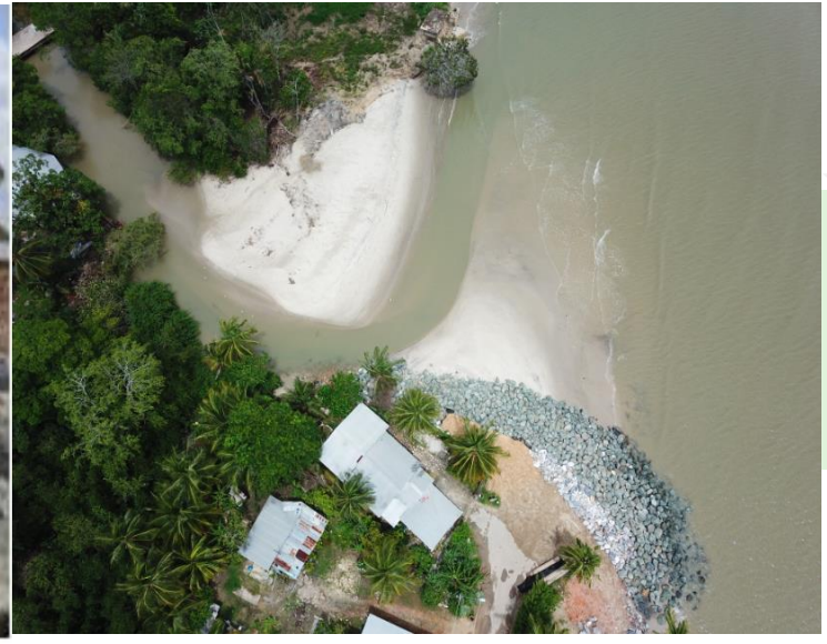
San Souci Shoreline Stabilization Works – 68% completed
