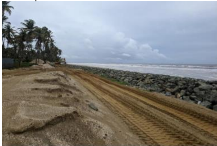
Cocos Bay Shoreline Stabilization Works- 84% completed
