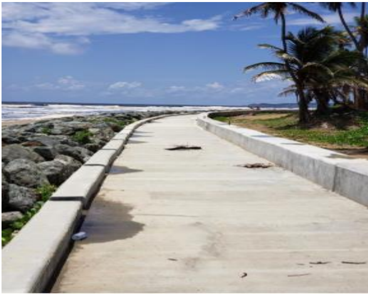
South Cocos Bay Shoreline Stabilization Works – 84% completed
