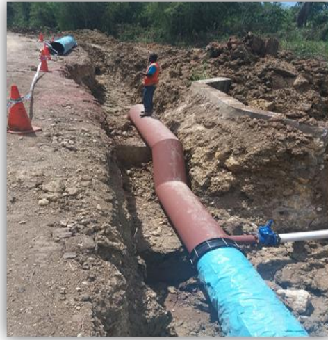
Installation of Main to the Union Industrial
