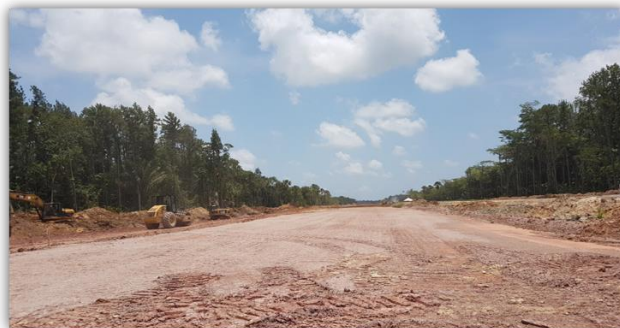
Spreading of Embankment Fill on both East and West Bound lanes of the Carriageway between 9+081-9+200
