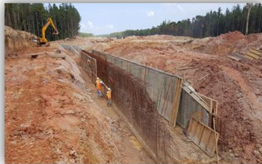
Box Culvert for the Connector Road
