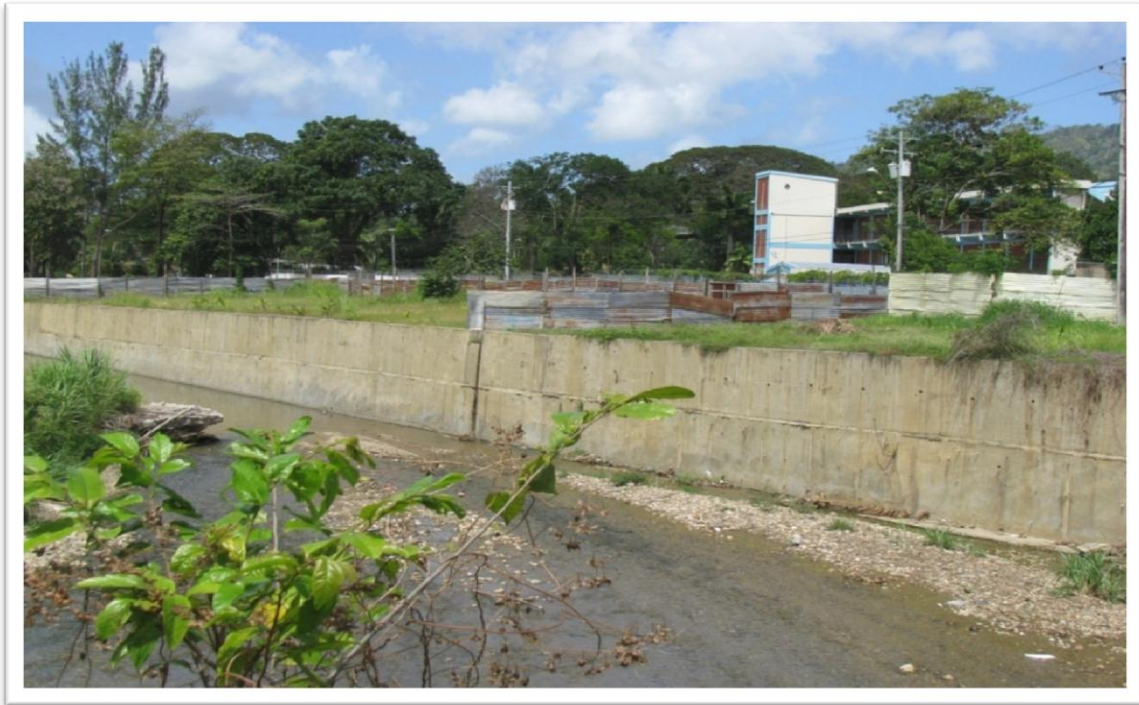
Reinforced concrete wall constructed on the St. Joseph River at Site 3 Farm Road
