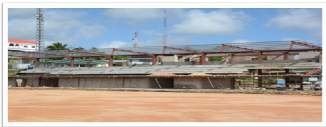
Yolande Pompey Recreation Facility Pavillion under construction
