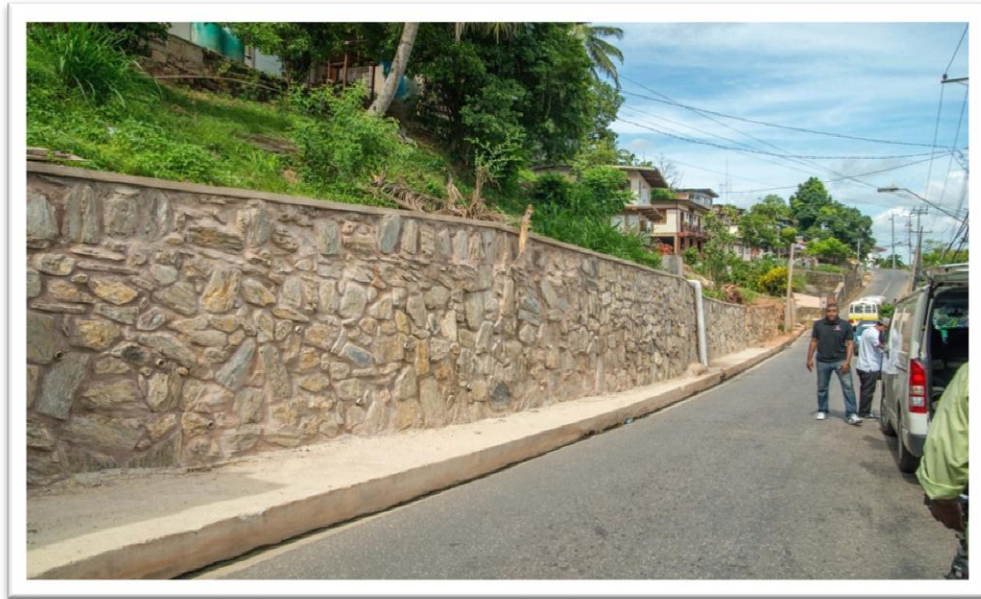
Retaining wall at Red Hill Morvant
