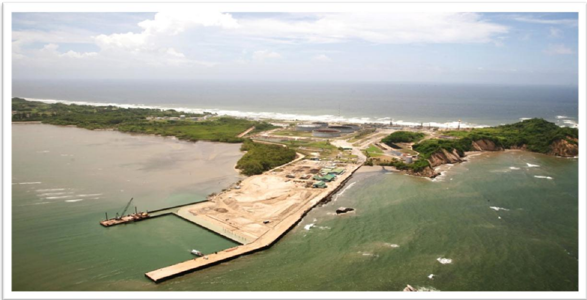
Overview of construction of the Galeota Port
