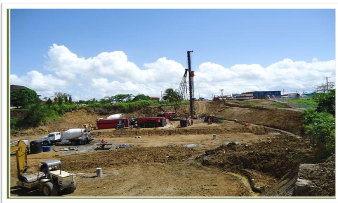
Construction works at B1/3 Calcutta Road No. 2
