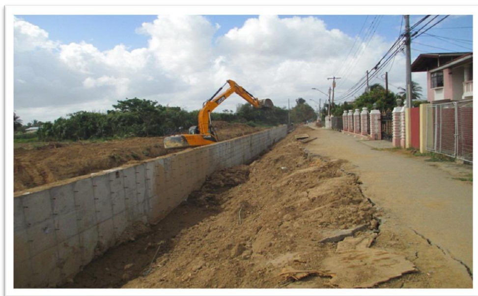
Tunapuna River Improvement Works – Dry River Trace
