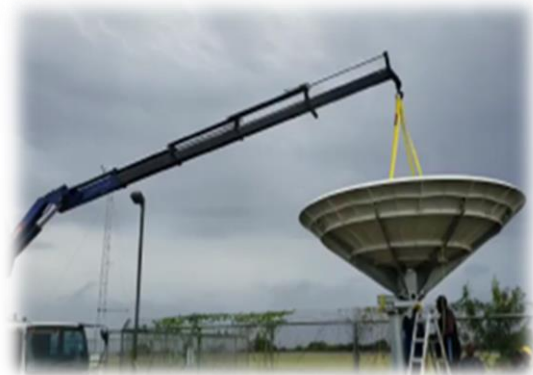
Installation of Ground Satellite Station Receiving Antenna
