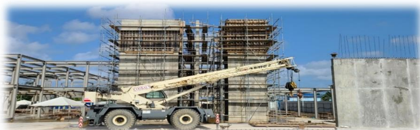
Shear Walls #13, #14 and #15 (Zone 4) Constructed, Structural Steel Columns and Beams Installed (Eastern view)
