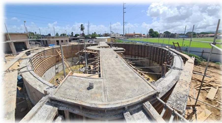
Aeration tank: Final concrete completed
