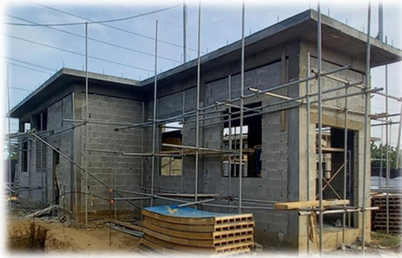
Sludge Treatment Building: Blockwork in progress
