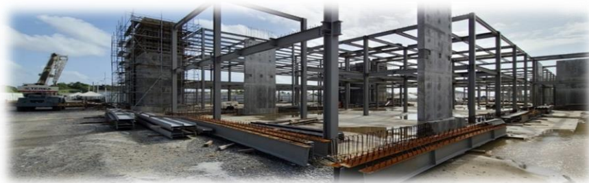
Sangre Grande Hospital, Shear Walls #4 and #23 (Zones 2 and 3) Constructed, Structural Steel Columns and Beams Installed (Western view)
