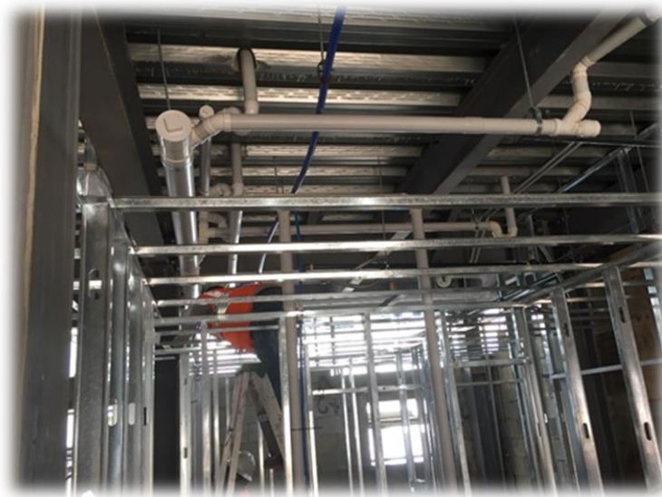
Plumbing Installation at the Josephine Shaw House
