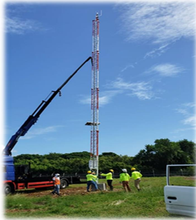
Erection of Low-Level Windshear Alerting System (LLWAS)
