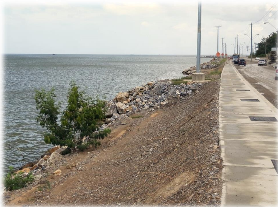
Coastal Works at San Fernando
