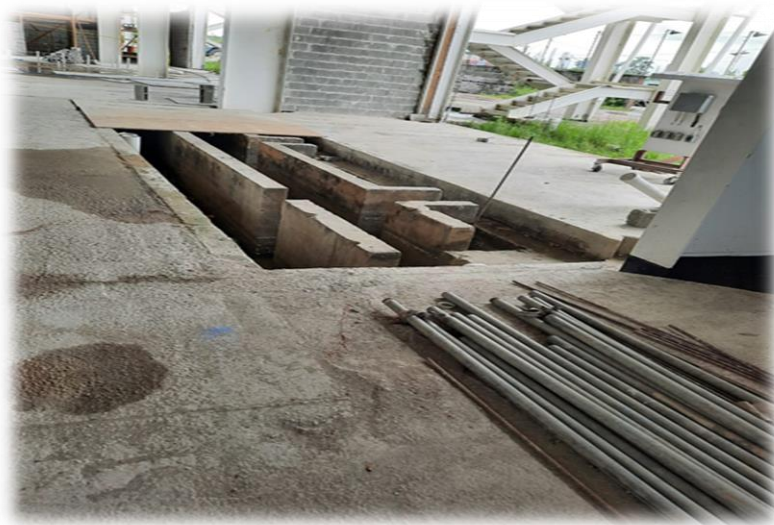
Ongoing works at Mahaica Oval
