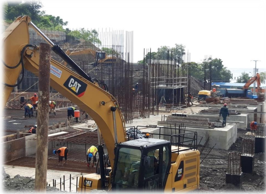
San Fernando General Hospital Car Park
