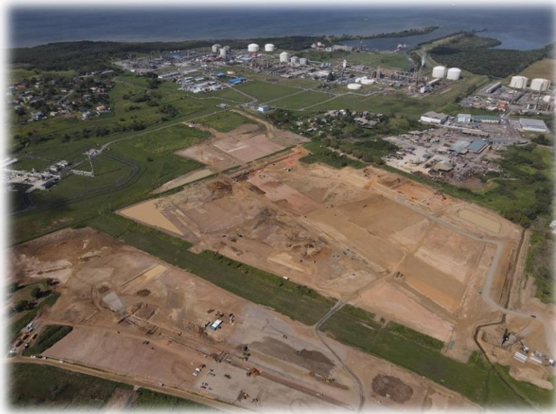
Aerial view of the Phoenix Park Industrial Estate Construction Site
