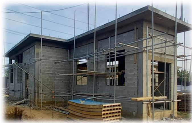
Sludge Treatment Building: Blockwork in progress
