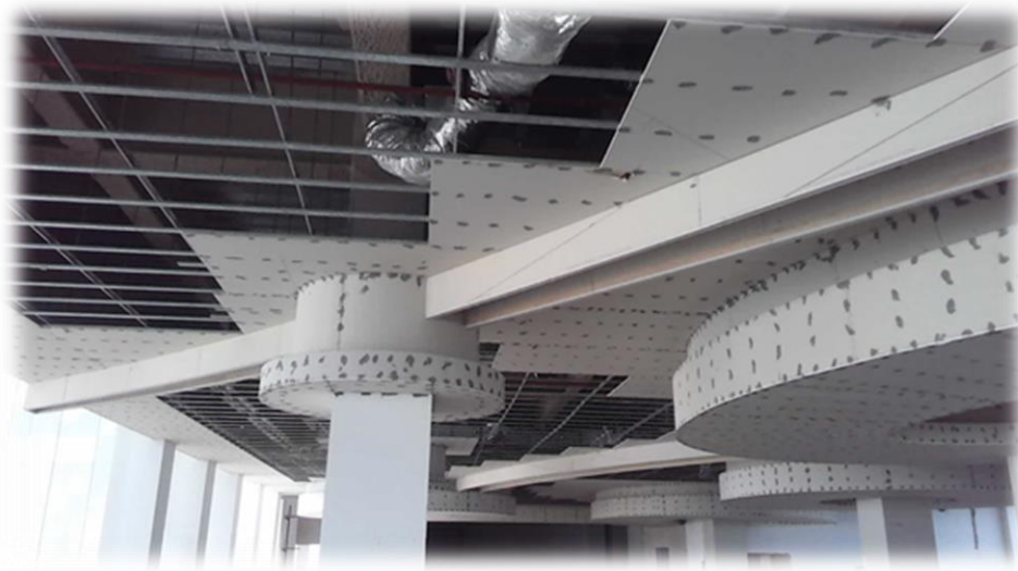
Air conditioning, ceiling, electrical work West Block
