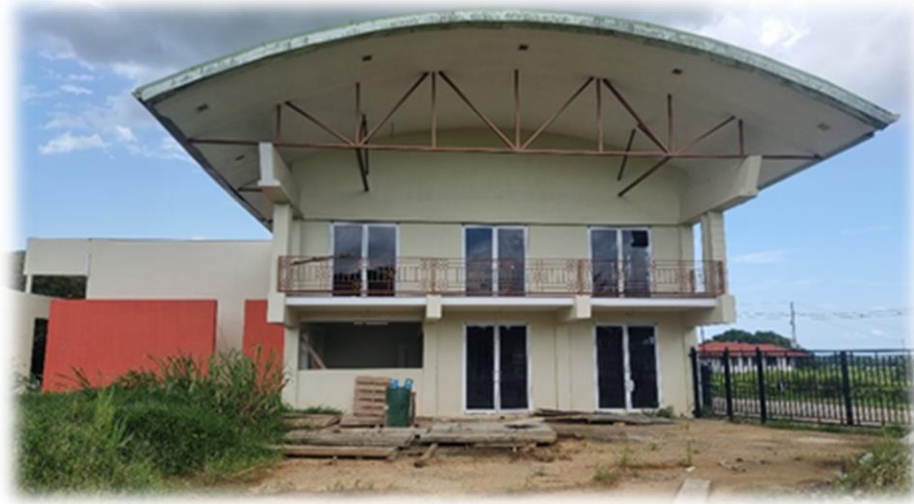
Ongoing works at Sevilla Club
