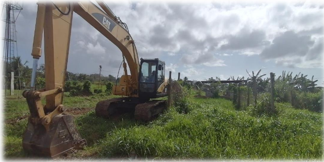
Clearing site for compost depot
