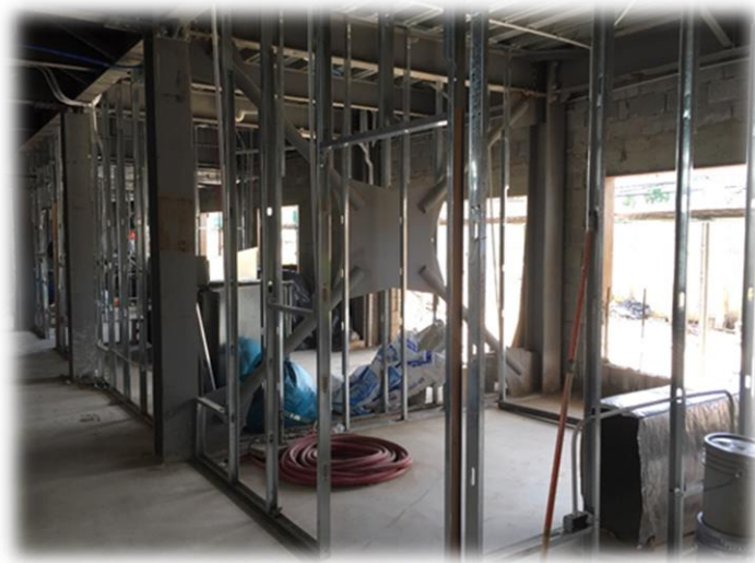
Wall Framing at the Josephine Shaw House
