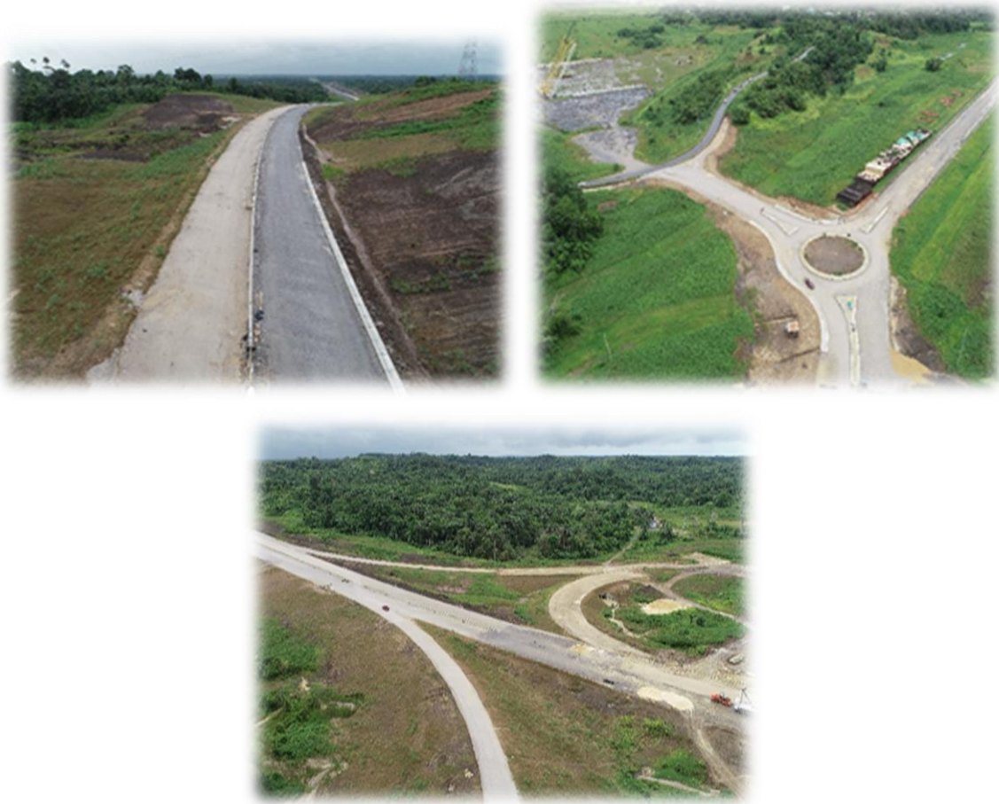
PACKAGE 5B- Completion of the SHHEPF Segment Between Eccles Trace and La Brea Top Right- Eccles Trace to La Brea Segment, Lower Left- SMR Roundabout, Lower Right-La Brea Connector
