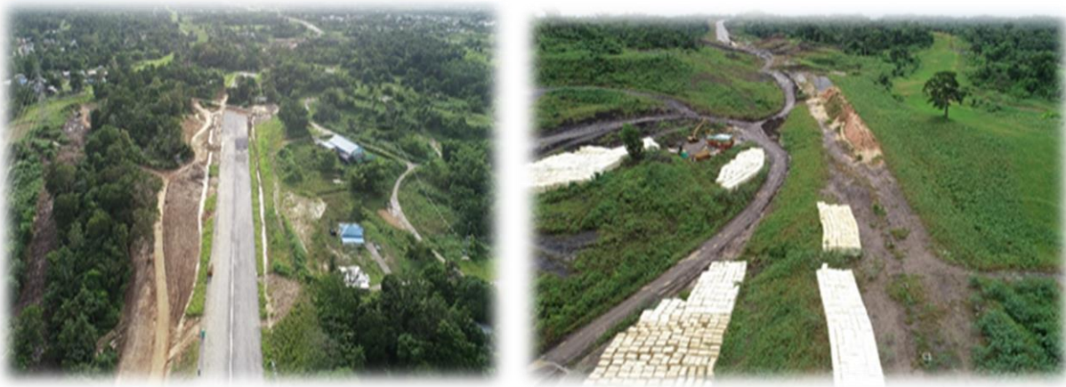
Package 6C - Completion of the segment between La Brea Interchange to Southern Main Road (B44) and from Fyzabad Road to the Mon Desir Interchange. Left- Fyzabad to Mon Desir, Right-La Brea to Southern Main Road
