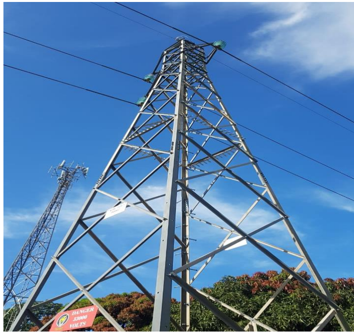
Refurbishment of the North Oropouche-Toco Link #1 33 kV Circuit
