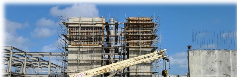
Sangre Grande Hospital, Shear Walls #4 and #23 (Zones 2 and 3) Constructed, Structural Steel Columns and Beams Installed (Western view)
