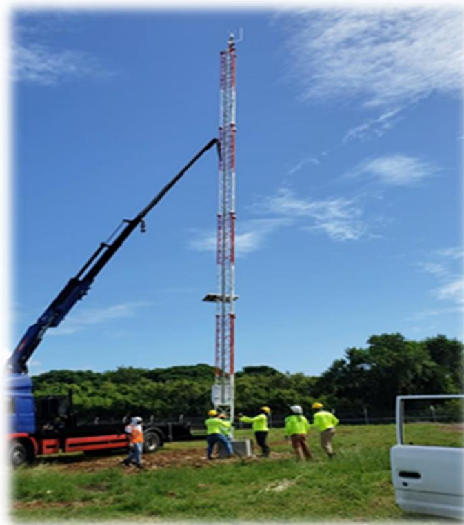
Erection of Low-Level Windshear Alerting System (LLWAS)
