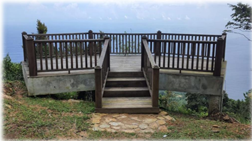
Observation Deck completed at Paramin Village Lookout
