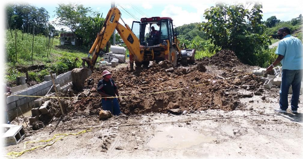
Ongoing works at Samlalsingh Trace
