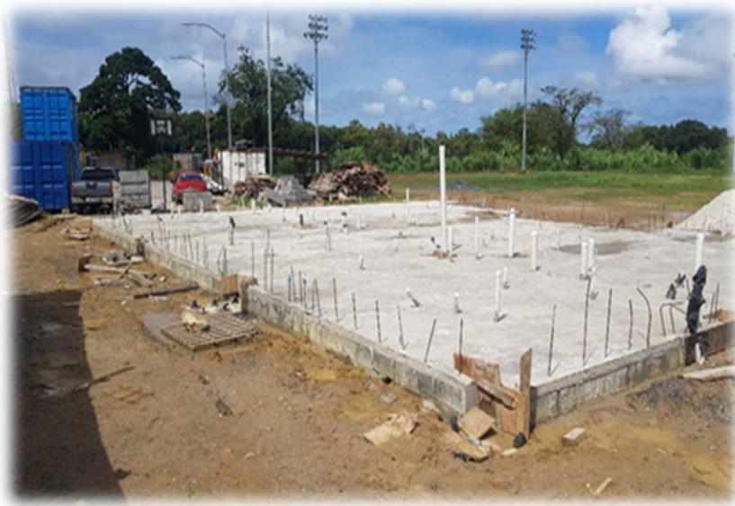
Ongoing works at Todd's Road Recreation Ground
