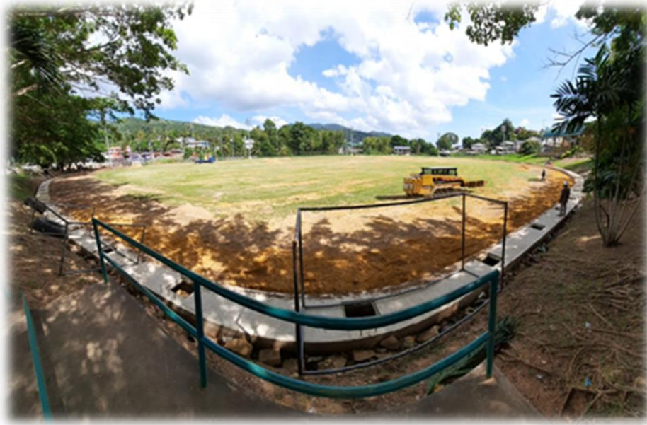
Works executed at Park Street Recreation Ground
