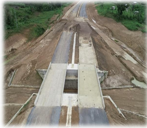
PACKAGE 1D-Completion of No. 8 Road Overpass and Guapo River Bridge (left)
