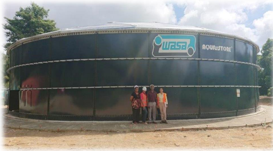
Installation of a three hundred thousand (300,000) IG tank at the Guanapo Water Treatment Plant
