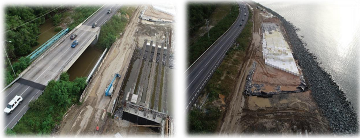
Package 5A - Completion of the segment between the Godineau River Bridge and the Mosquito Creek Bridge of the SHHEPF.
