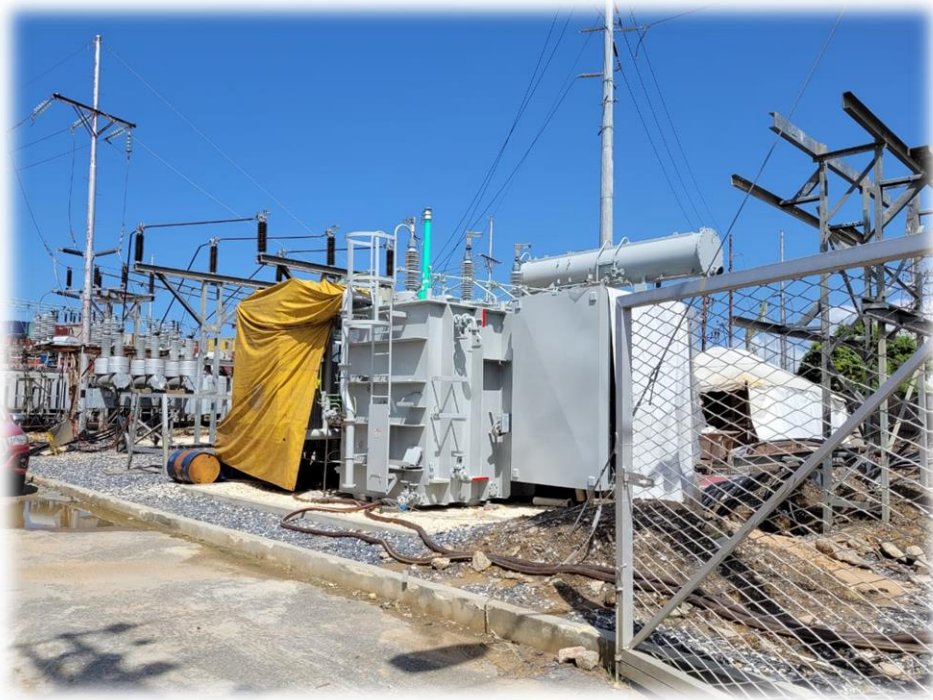
Installation of new transformer at Wrightson Road Substation
