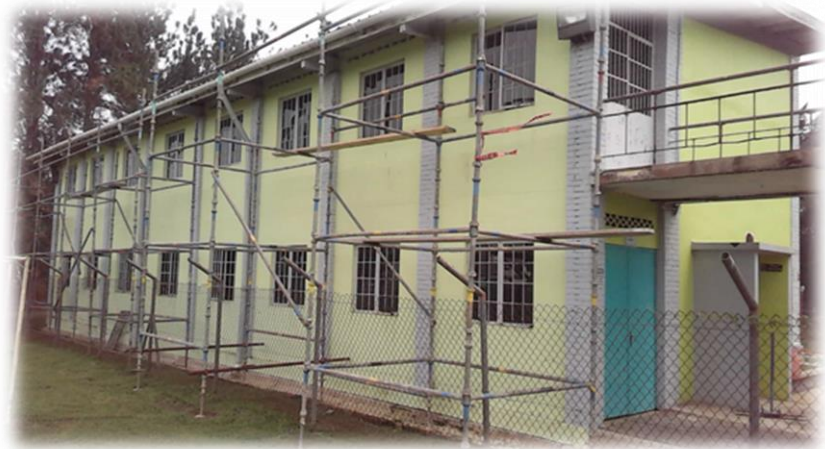
Roofing, ceiling and interior works completed on student residence
