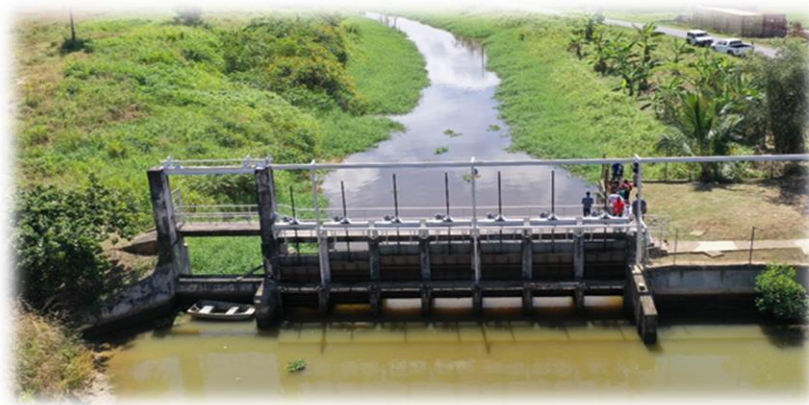
Gate Structure at St John's (Fyzabad)
