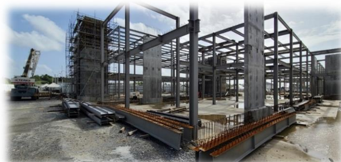
Sangre Grande Hospital, Shear Walls #4 and #23 (Zones 2 and 3) Constructed, Structural Steel Columns and Beams Installed (Western view)
