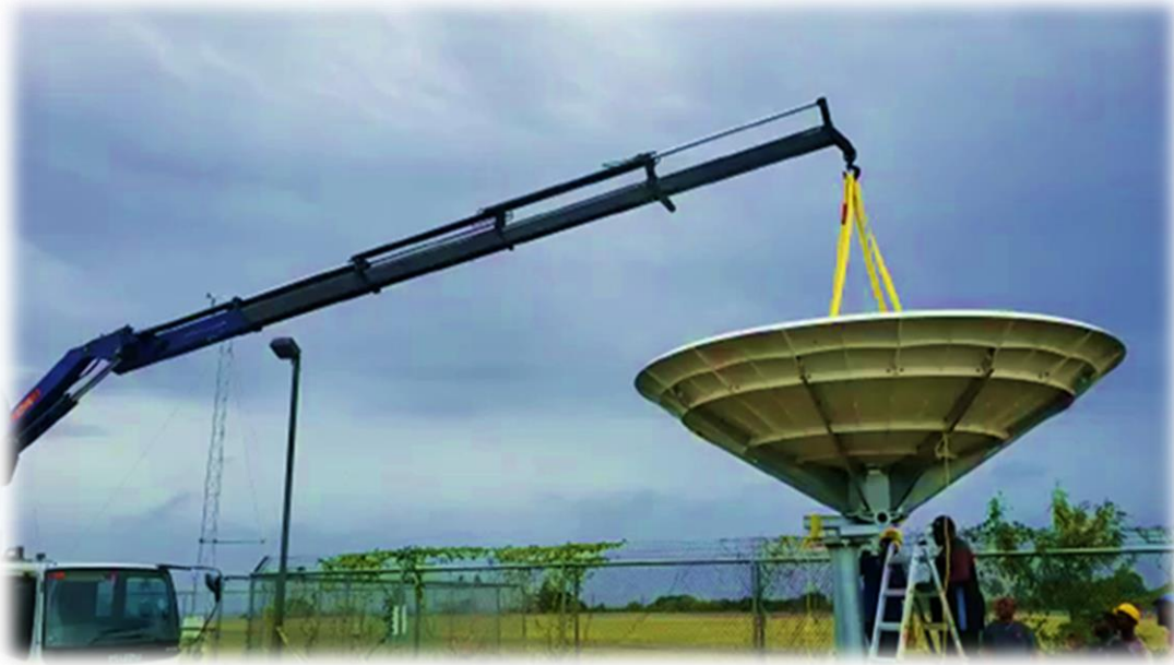
Geostationary Operational Environmental Satellite (G.O.E.S) Ground Station Satellite Dish
