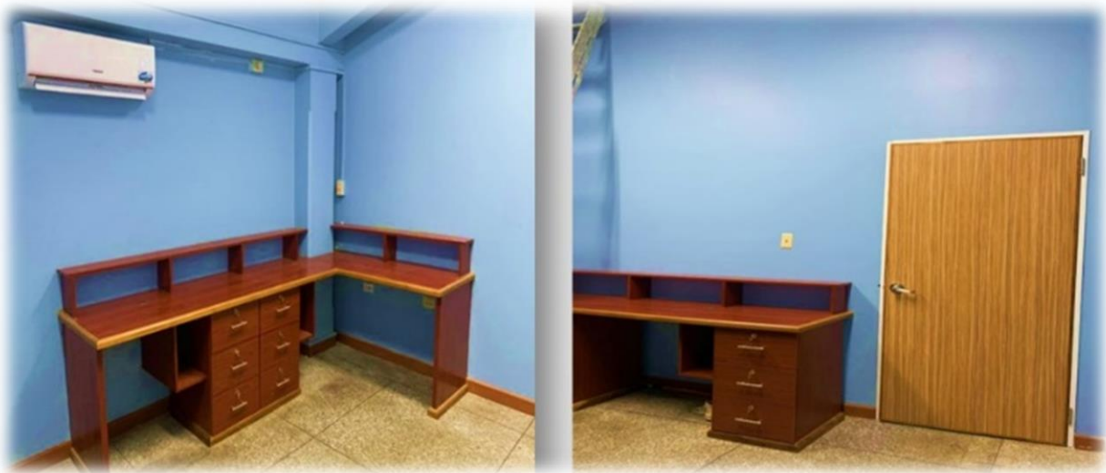
Remodeling of spaces to facilitate CCTV and supporting staff at Sangre Grande- 90 percent completed
