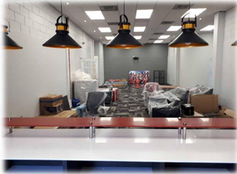
Ongoing works at Dwight Yorke Stadium
