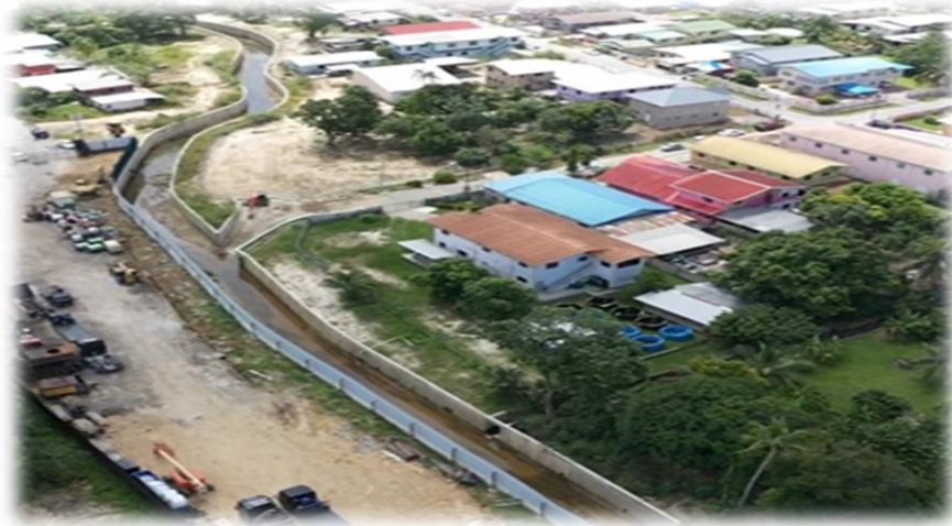
Drainage Works on Diana River (Chase Village)
