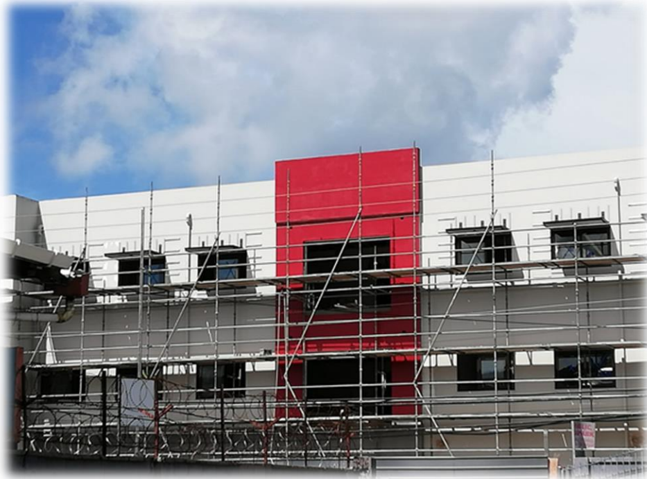
Ongoing works at the Josephine Shaw House
