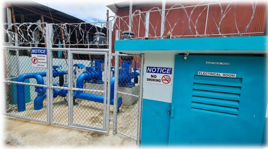
Refurbishment of Richplain booster pumping station
