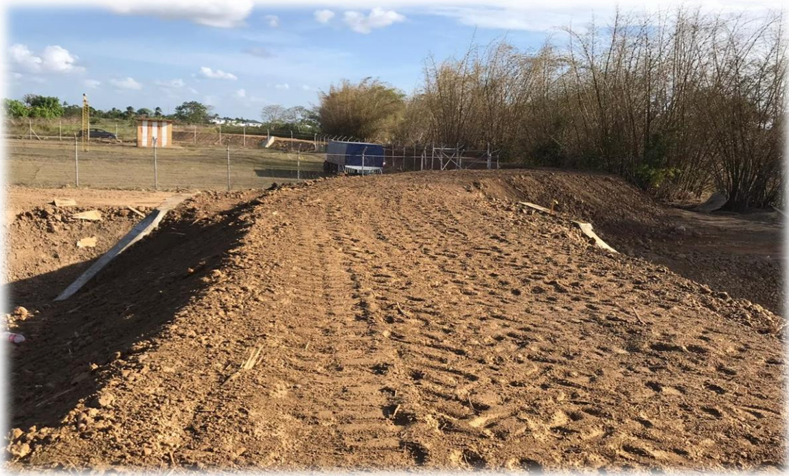
Embankment Works on the Caroni River
