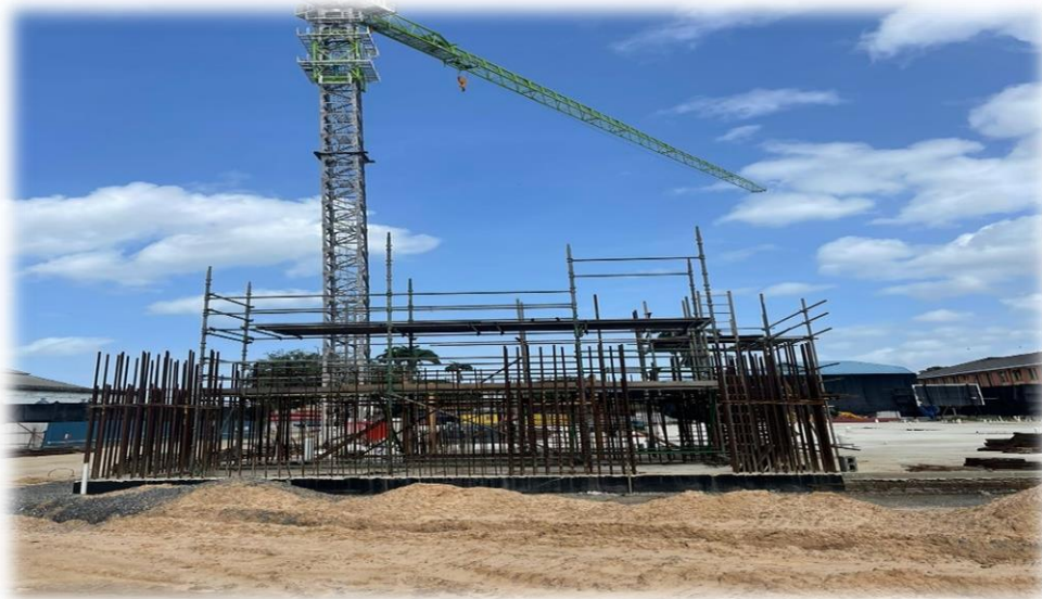
Ground Floor Slab Installed (Eastern view), Shear Wall 20-23 Rebar Installation
