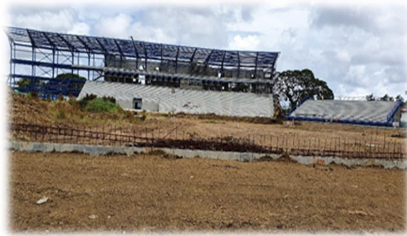
Ongoing works at Skinner Park
