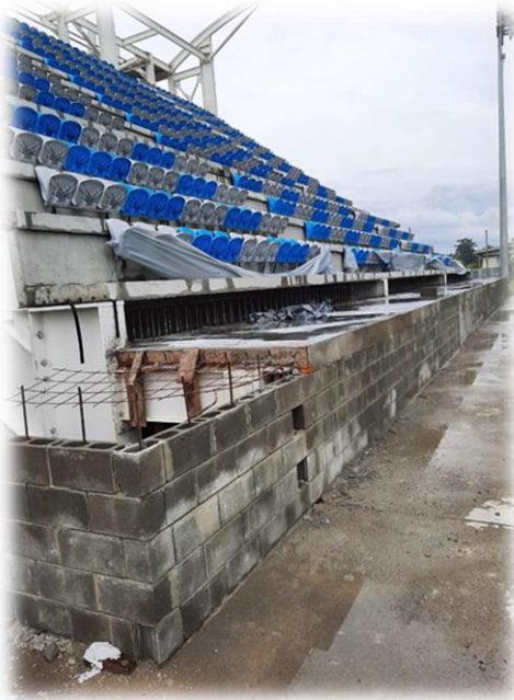
Ongoing works at Mahaica Oval
