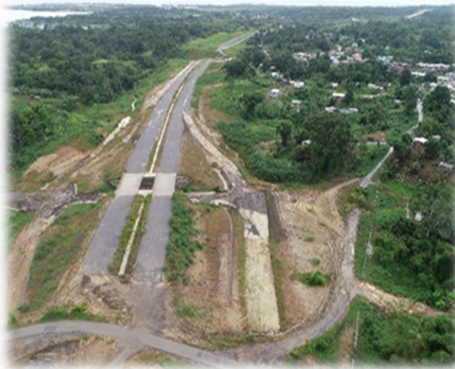
Package 5D - Completion of the segment between Southern Main Road (B44) to Dunlop Roundabout of the SHHEPF
