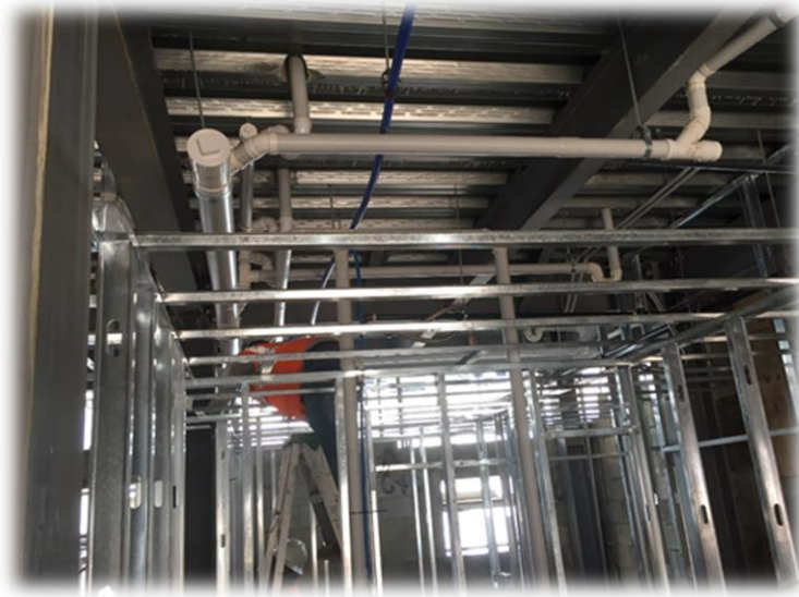
Plumbing Installation at the Josephine Shaw House
