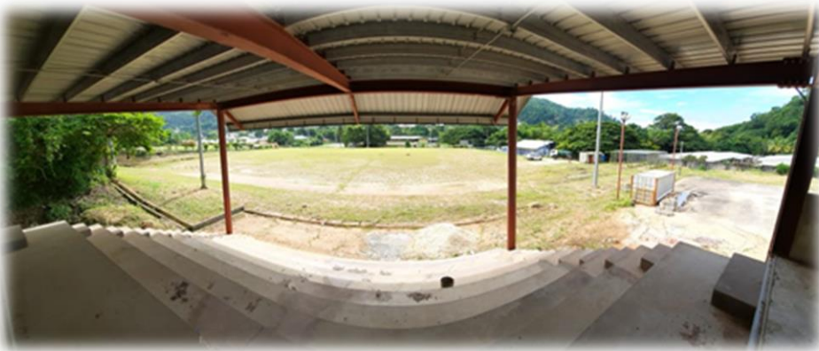
Ongoing works at Bourg Mulatresse Recreation Ground
