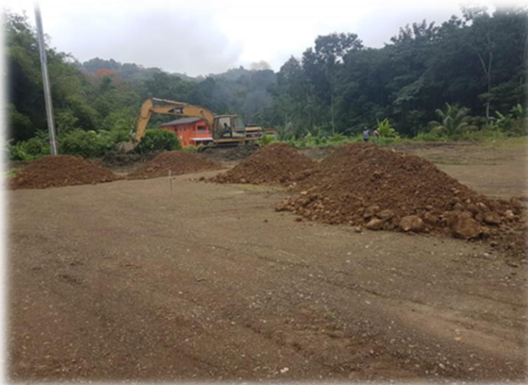
Ongoing works at Grand Riviere Recreation Ground
