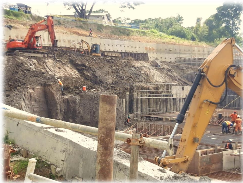
San Fernando General Hospital Car Park
