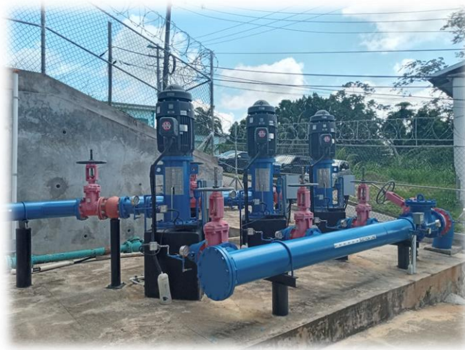
Installation of a polyvinyl chloride (PVC) main pipeline from Calvary Hill Booster to Calvary Hill Reservoir
