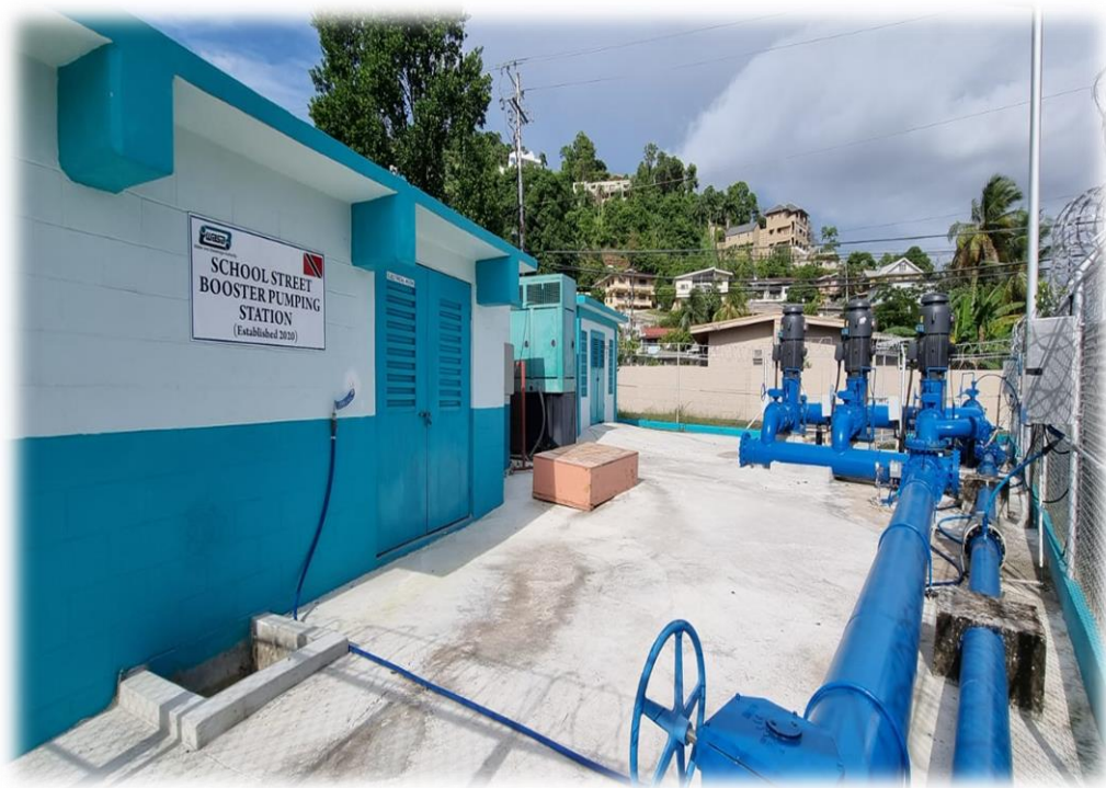
Refurbishment of School Street booster pumping station
