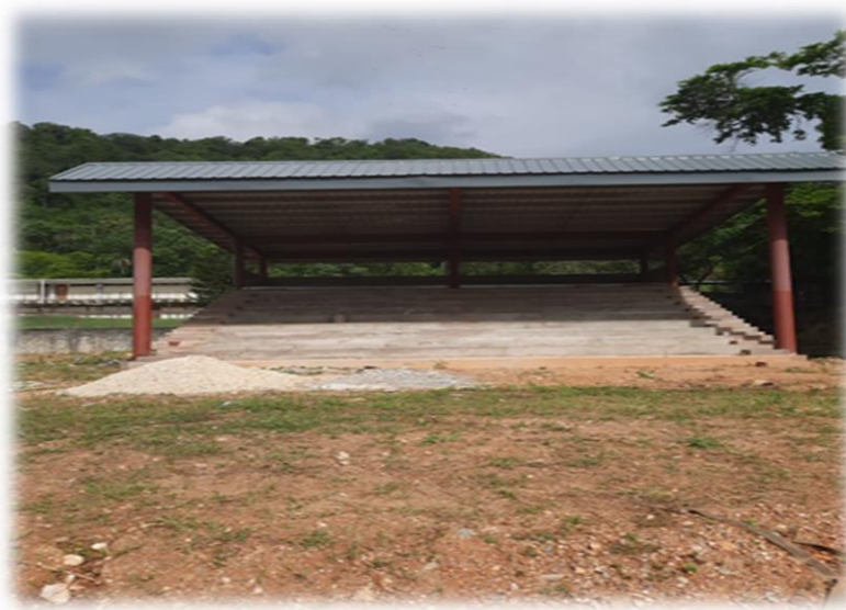
Ongoing works at Bourg Mulatresse Recreation Ground
