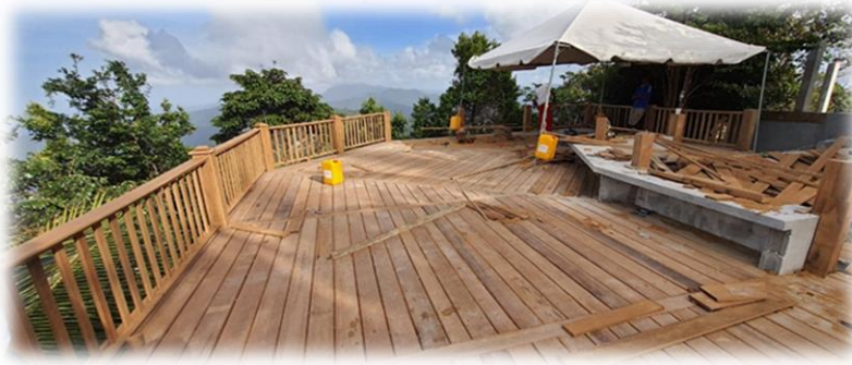
Ongoing works at Paramin Village Lookout
