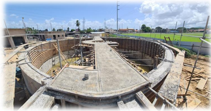
Aeration tank: Final concrete completed
