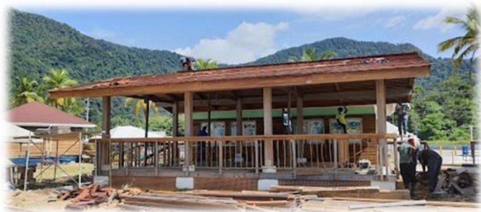
Ongoing works at Maracas Beach Facility
