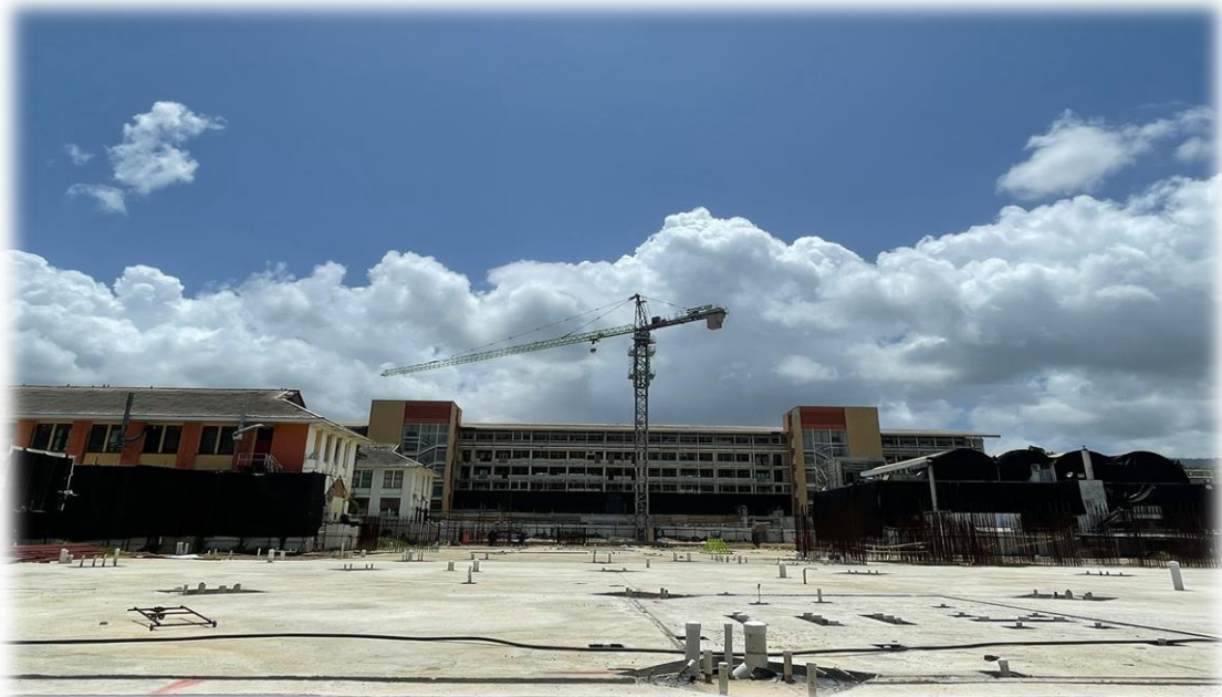
Central Block, POSGH - Ground Floor Slab Installed (Southern view)
