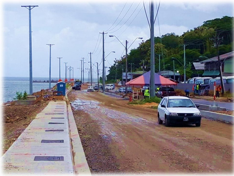
Dualling of Lady Hailes Avenue at PTSC Compound
