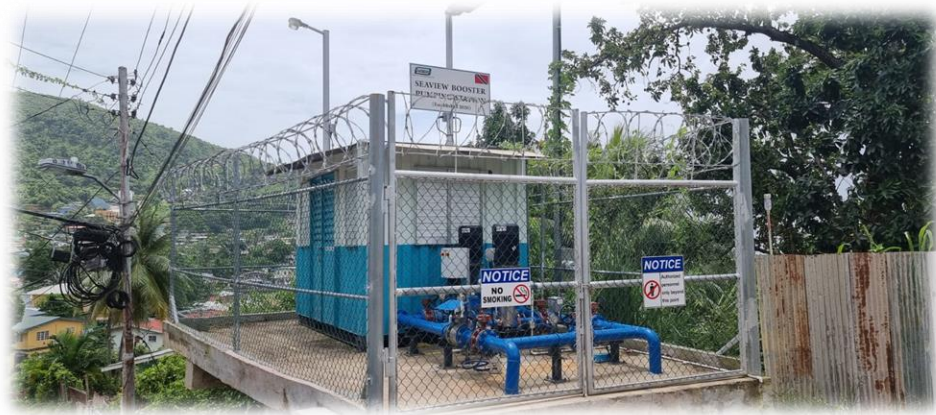
Construction of Seaview booster pumping station
