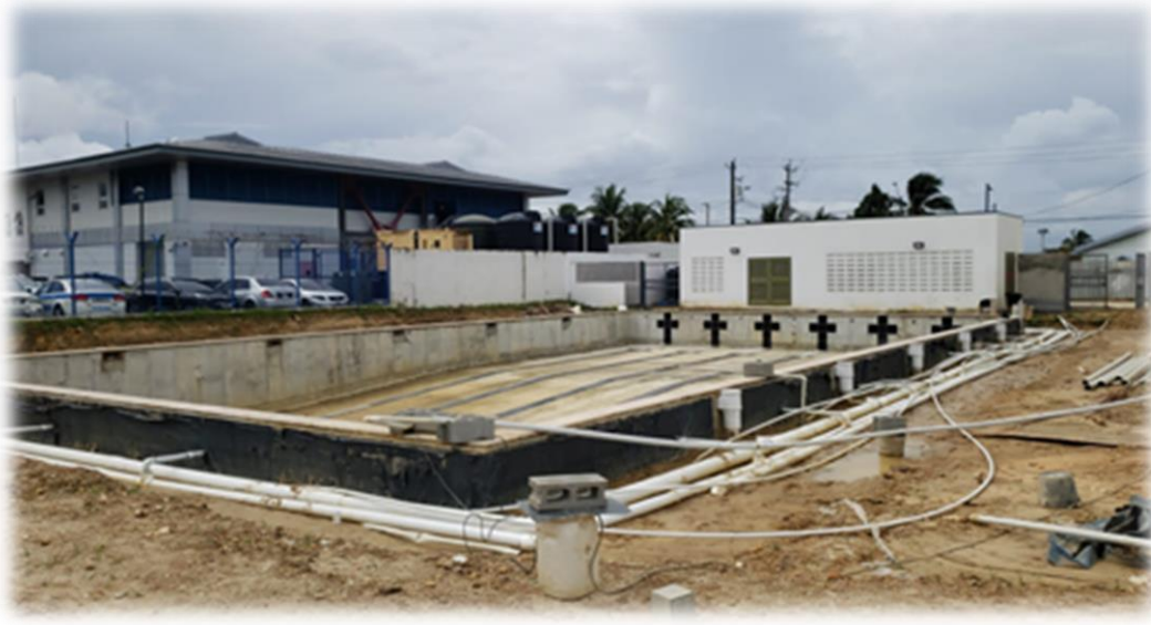
Ongoing works at Maloney Community Swimming Pool
