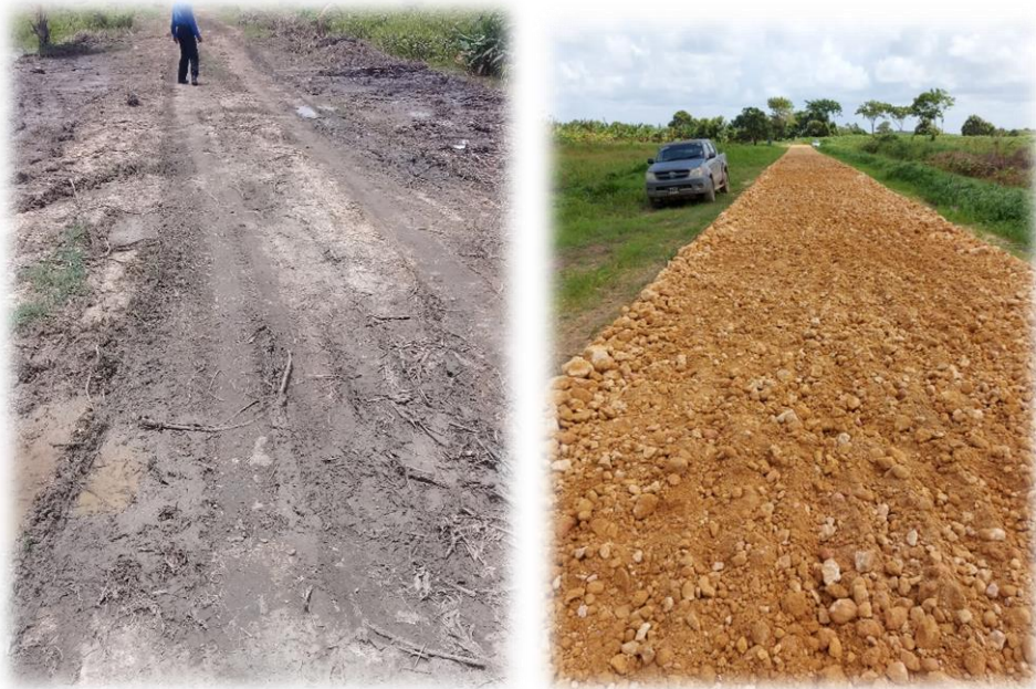
Rehabilitation of Roadway at Orange Grove
