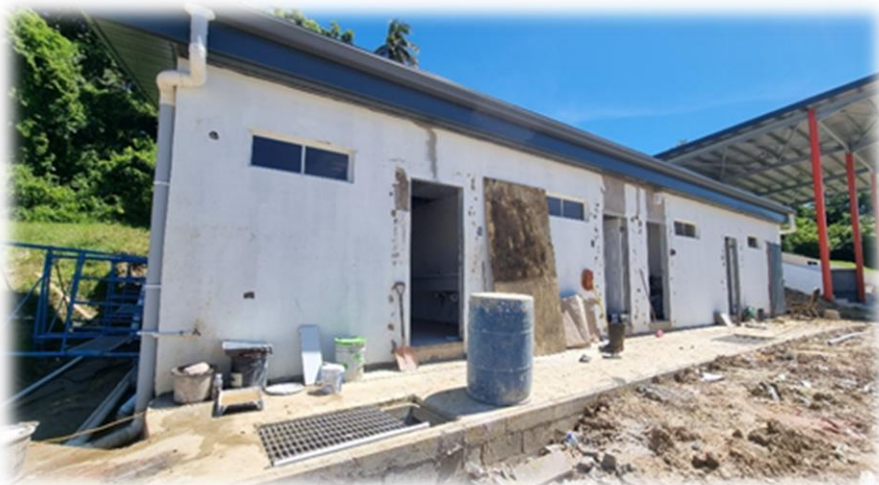
Ongoing works at Marac Recreation Ground
