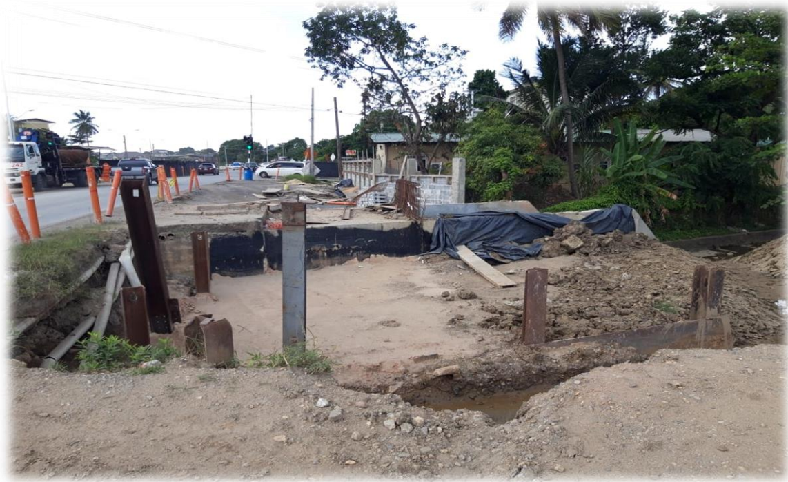
Bridge Works at Lady Hailes Avenue near Embacadere
