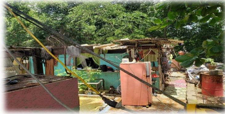
Homes of Families Identified for Assistance by the Housing Village and Improvement Programme
