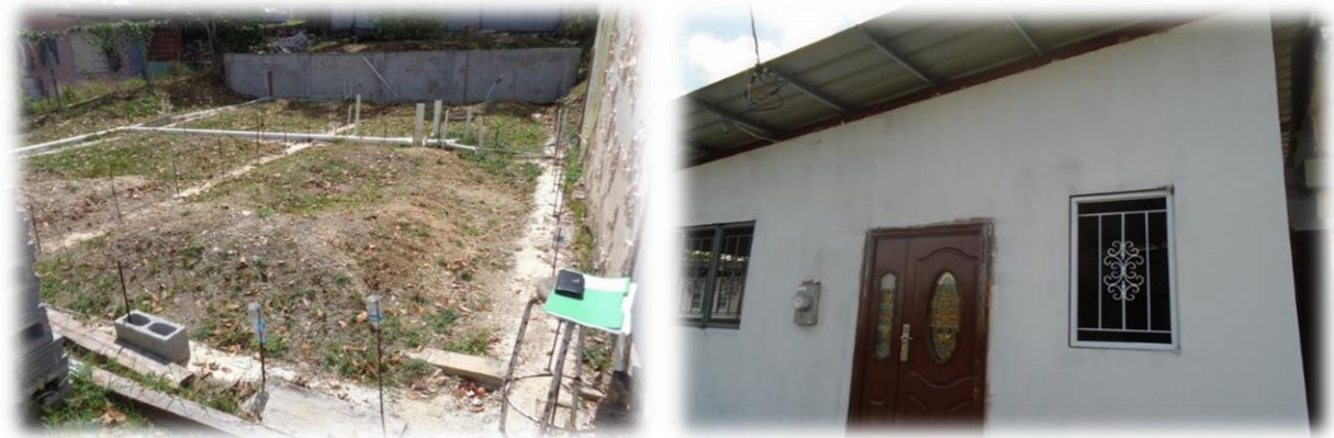
Housing and Improvement Grant Before and After Home Construction
