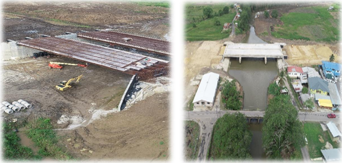
Package 1B -Completion of the Mon Desir Interchange Bridge and Oropouche River Bridge Photos showing Mon Desir Interchange Bridge (left) and Oropouche River Bridge (right)
