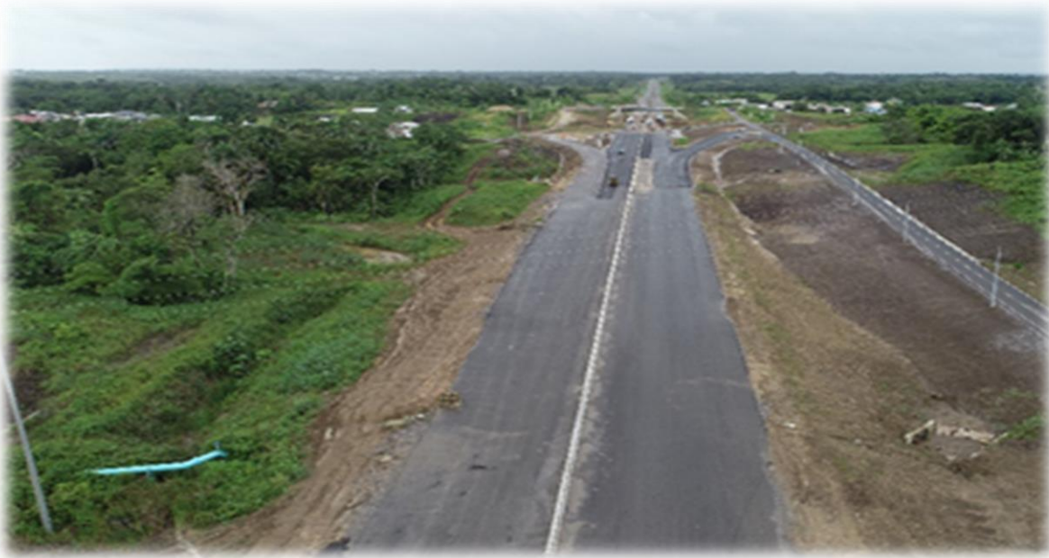
Package 2C - Completion of Mon Desir to Eccles Trace and St. Mary's Junction to Mon Desir Photo showing a segment of the Eccles Trace to Grants Road segment
