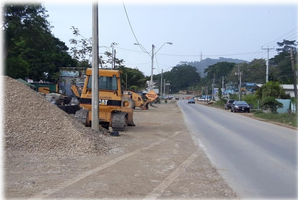
Dualling of Lady Hailes Avenue near entrance to San Fernando General Hospital
