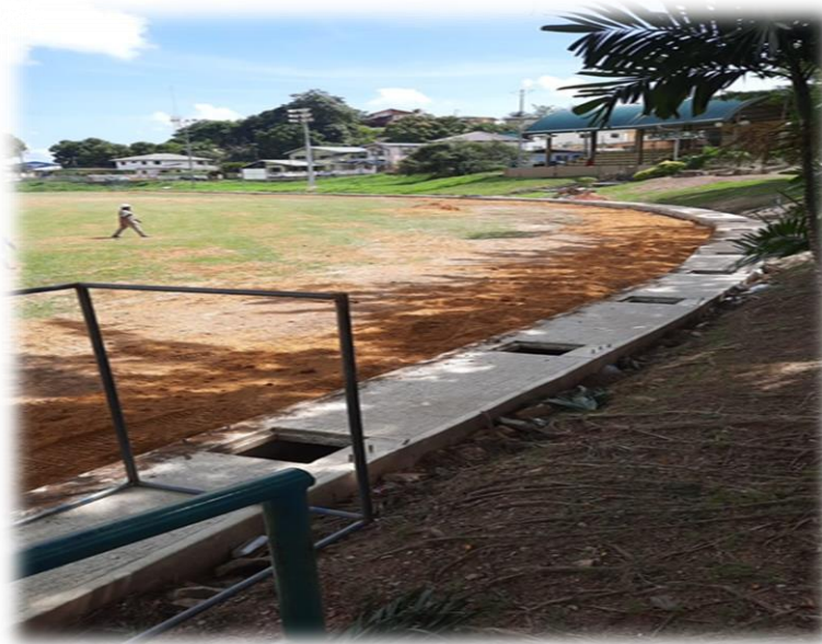
Ongoing works at Park Street Recreation Ground
