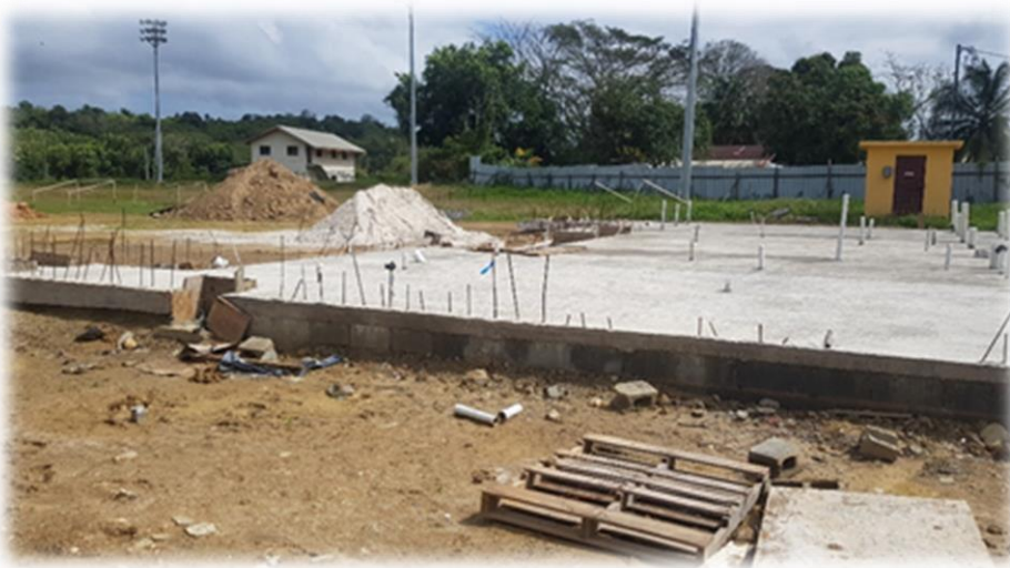
Foundation works done at Todd's Road Recreation Ground
