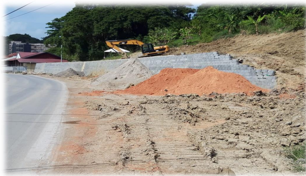
Construction of wall at beginning of Lady Hailes Avenue, San Fernando
