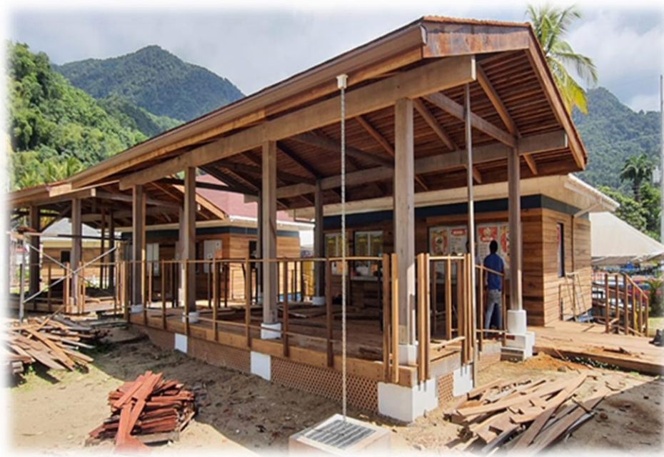
Ongoing works at Maracas Beach Facility
