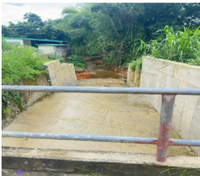
Construction of reinforced concrete U-Section at Bagatelle Diego Martin
