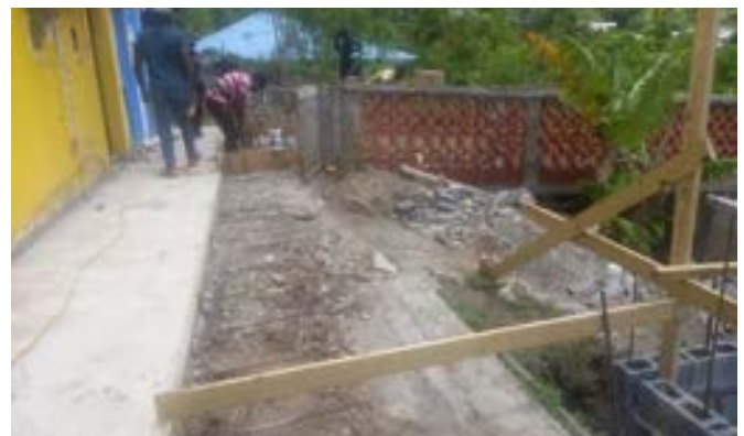
Court yard being prepared for casting
