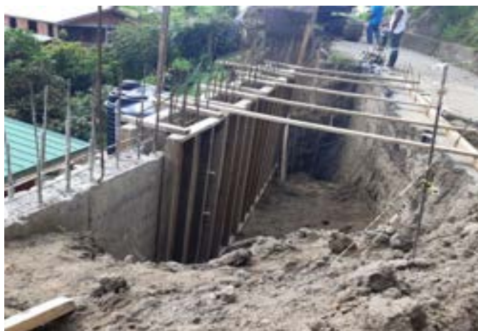
Retaining wall under construction at Runnemedede Village Street
